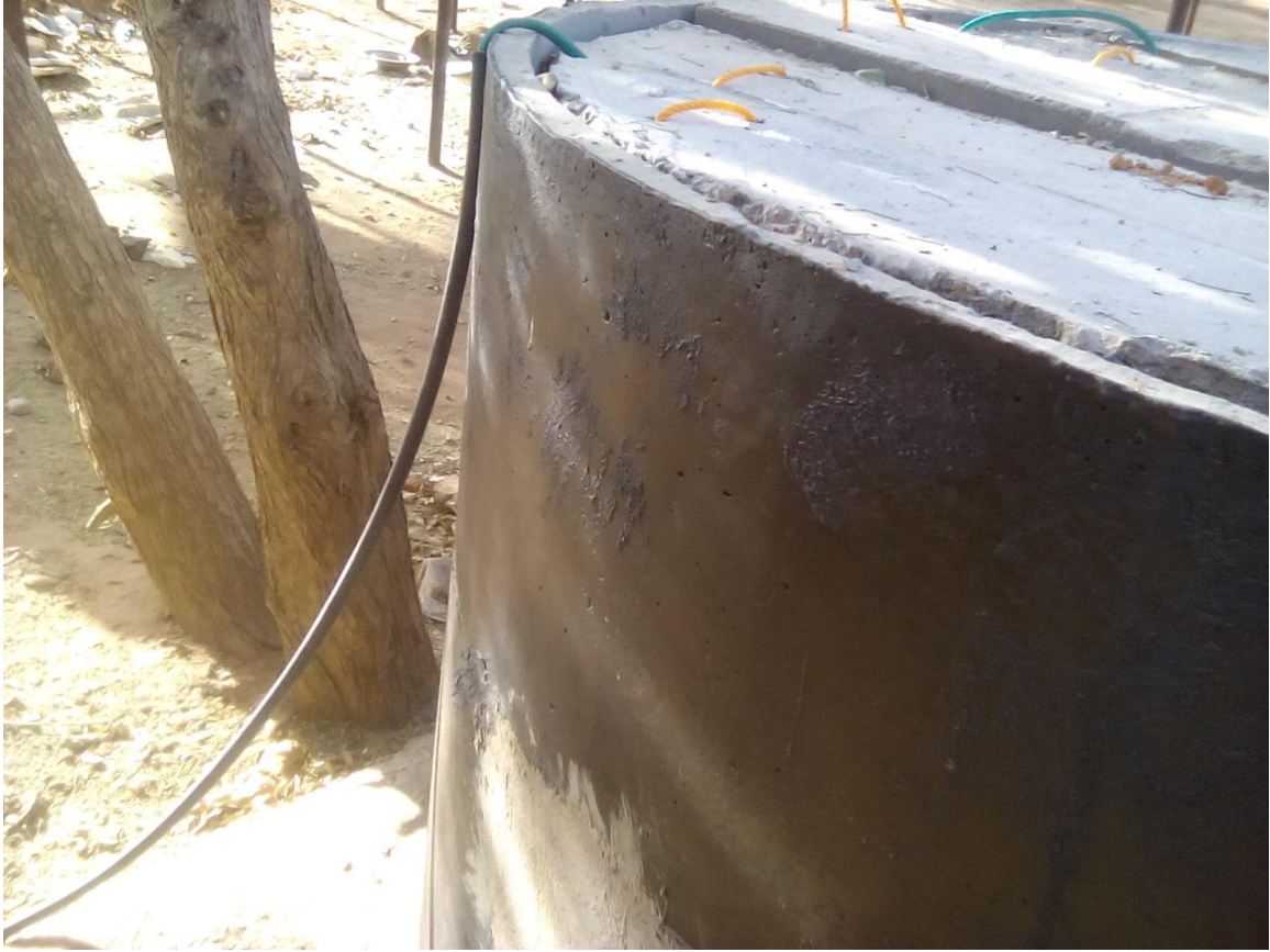
Biogas tube in side protection tube
