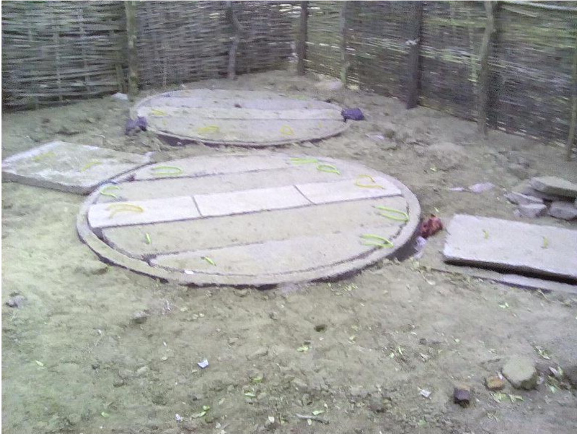
Main biogas digester & slurry storage tank
