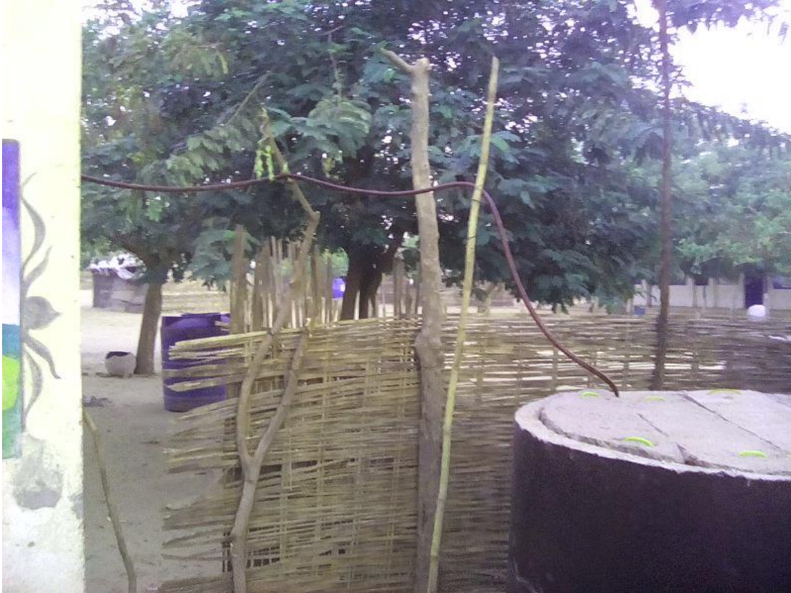
Biogas tube in side protection tube
